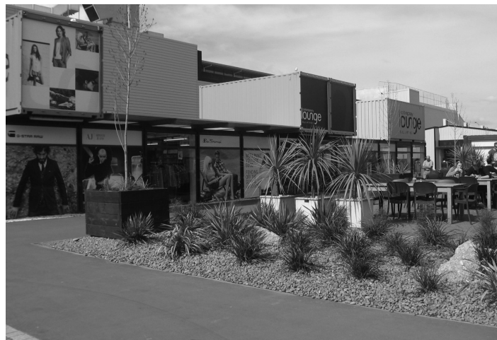
Re-Start Mall, Christchurch
